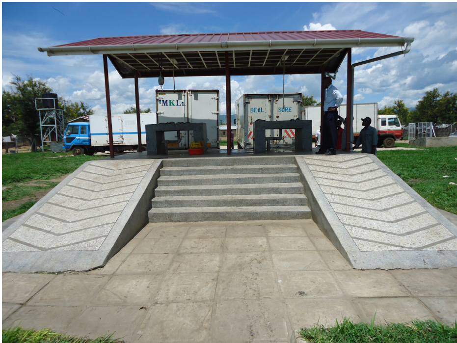
Improved clean water and sanitation facilities established at Kanala landing site in Ntoroko District, with support from QAFMP
