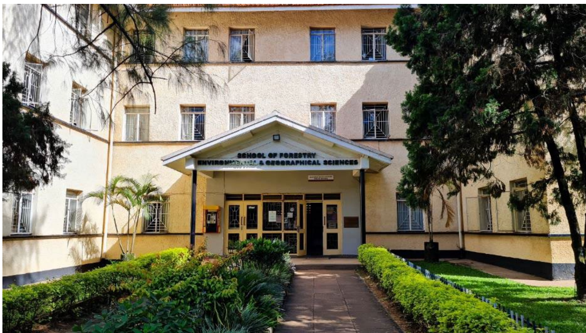
Photo 53: Entrance of the School of Forestry, Environmental and Geographical Sciences of Makerere University, Kampala, Uganda.
