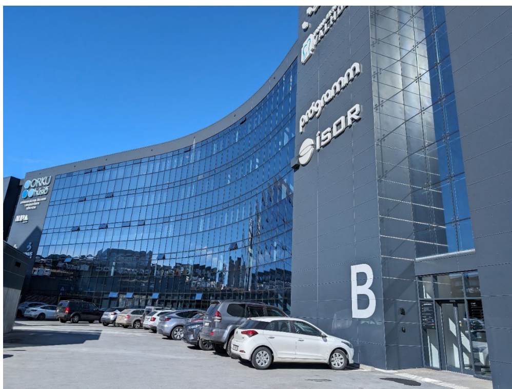
Photo 32: ÍSOR Building in Iceland, 15 April 2024
