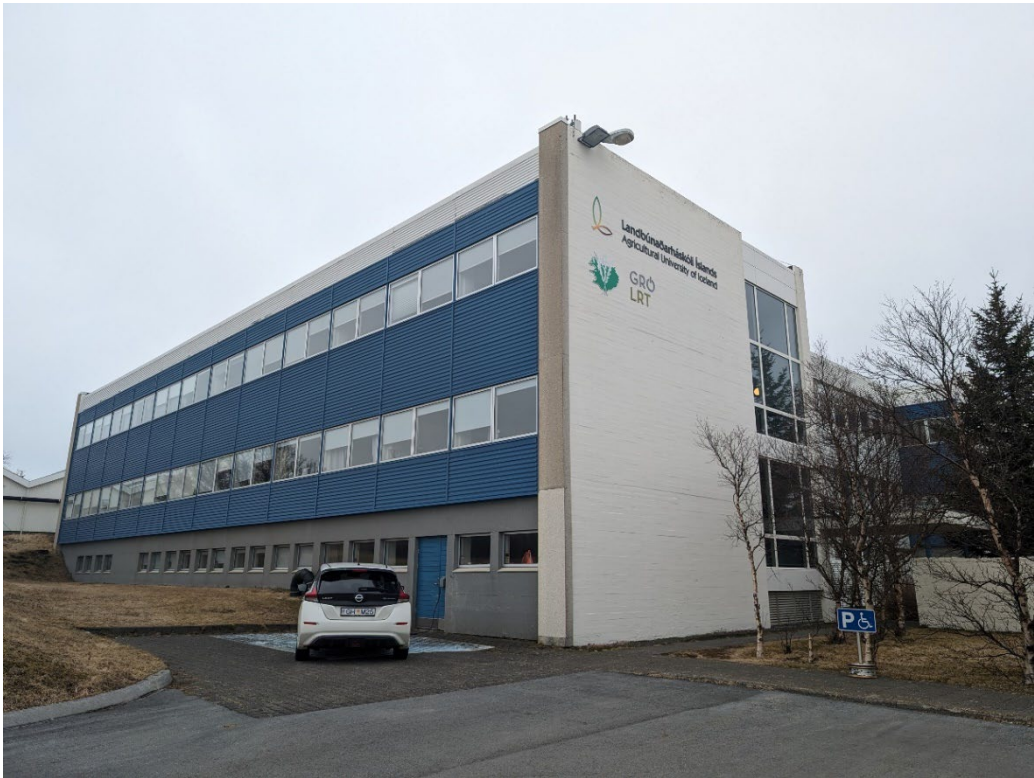
Photo 50: Building of the LBHÍ Branded with GRÓ LRT, 19 April 2024
