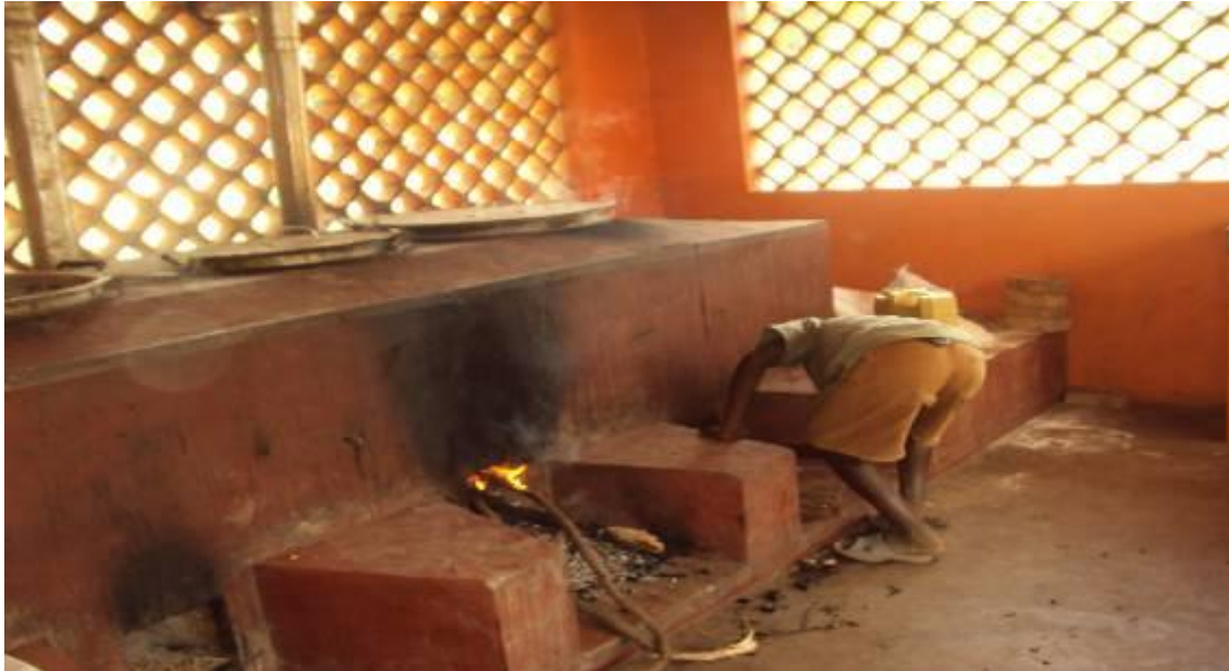
Photo 7: The newly constructed kitchen and its fuel saving stove at Bugoma primary school
