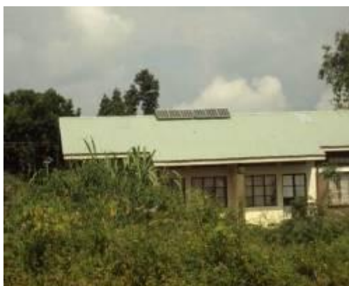
Photo 12: Staff quarters at Bukasa H/C With solar panels
