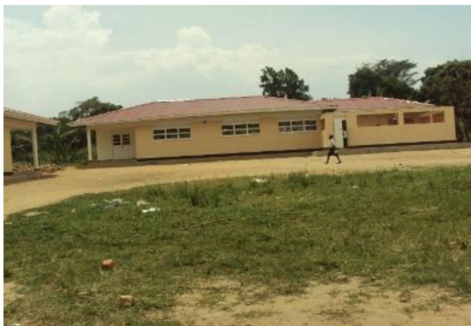
Photo 10: The New boys' dormitory block in Bugoma P/s
