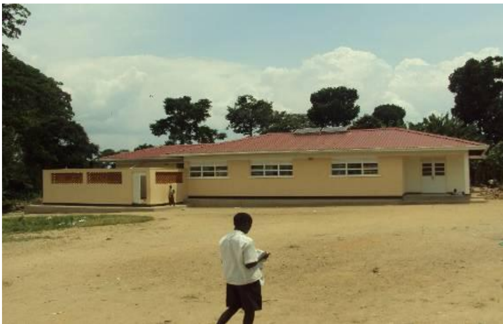
Photo 6: the constructed girls' dormitory at Bugoma Primary School
